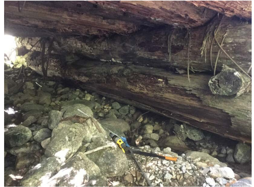
Left Bank Abutment when facing downstream
