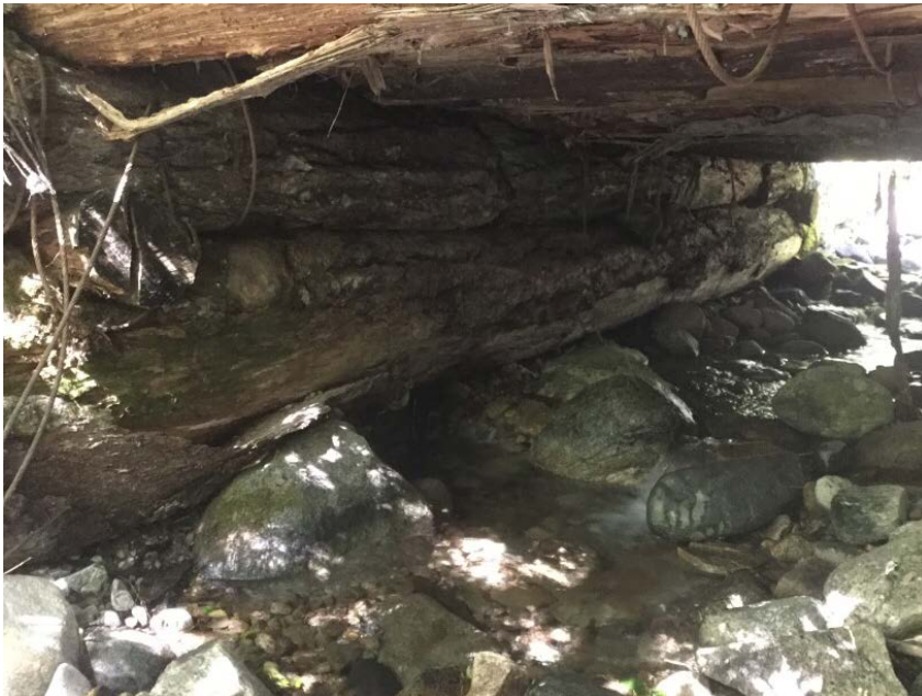
Right Bank Abutment when facing downstream
